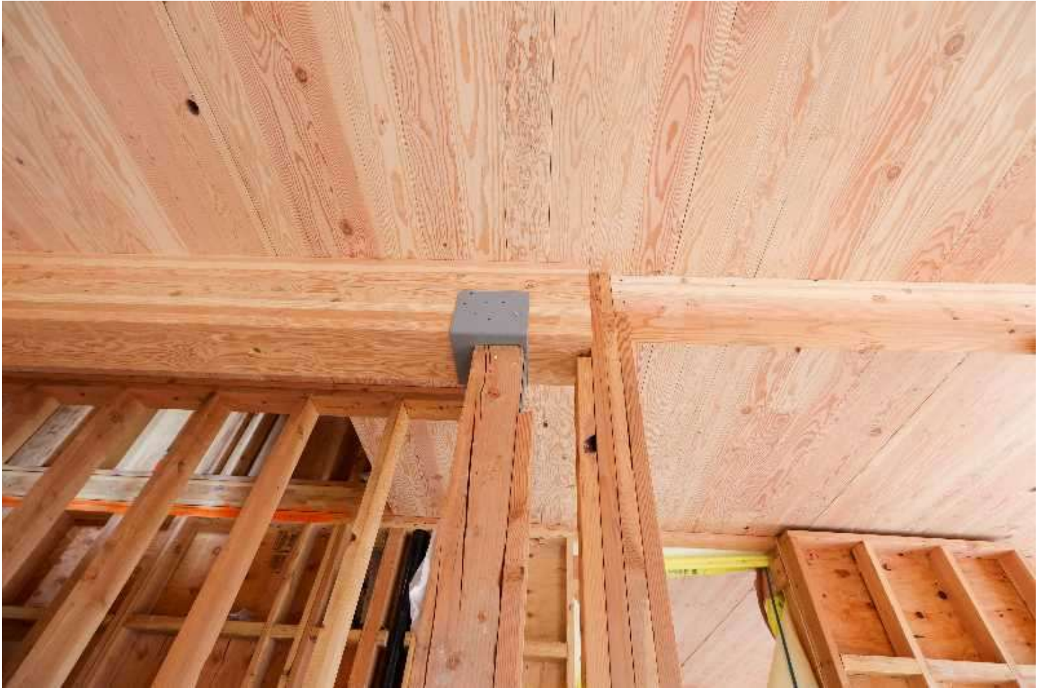
PMG PHOTO: JONATHAN VILLAGOMEZ - The Wilson Forest Park Townhomes Northwest use cross-laminated timber panels as flooring, and can be added to as a family grows like an east coast rowhome.
