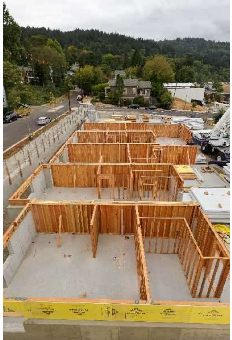
PMG PHOTO: JONATHAN VILLAGOMEZ - Some of the Wilson Forest Park Townhomes in Northwest Portland that have yet to reach full height. Forest Park is in the background..
