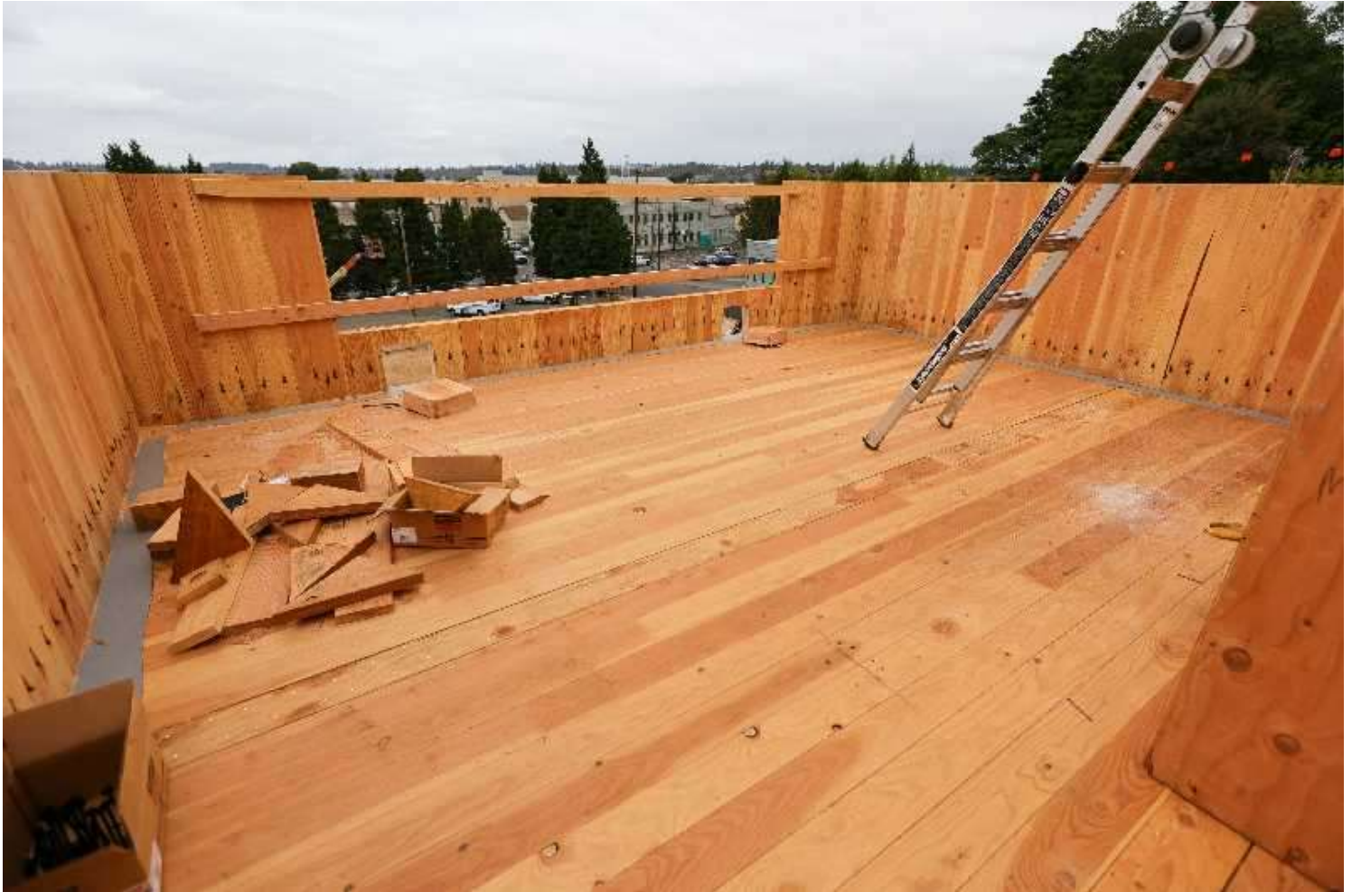
PMG PHOTO: JONATHAN VILLAGOMEZ - The Wilson Forest Park Townhomes Northwest with a view north over the industrial zone. The seven figure homes are in the next cool mixed-industrial according to developer Noel Johnson.
